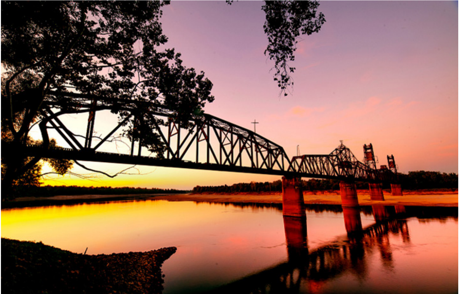
Yancopin Bridge, Desha County, AR. Photo courtesy Arkansas Department of Parks, Heritage and Tourism https://www.arkansas.gov
